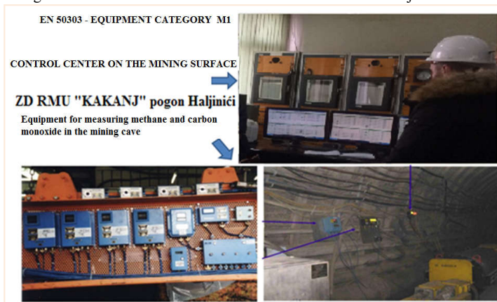
Figure 2. Information-communication infrastructure in Kakanj Coal Mine
